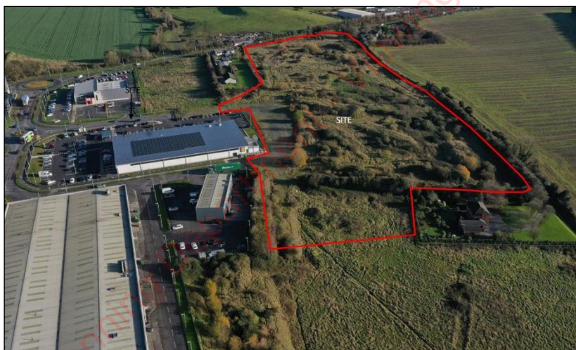
Figure 2 View of proposed development lands, with site outline in red, facing southeast (MCA Architects)
